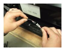
Route the cable inside the IPT securing it where necessary. Make sure there is a drip loop and that the connector is above the lowest point in the cabling.
